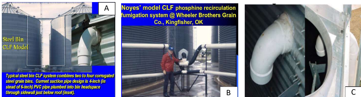
Fig. 1. First CLF model (A), caulked suction pipe elbows (B), CLF upper suction, lower pressure pipes (C).
