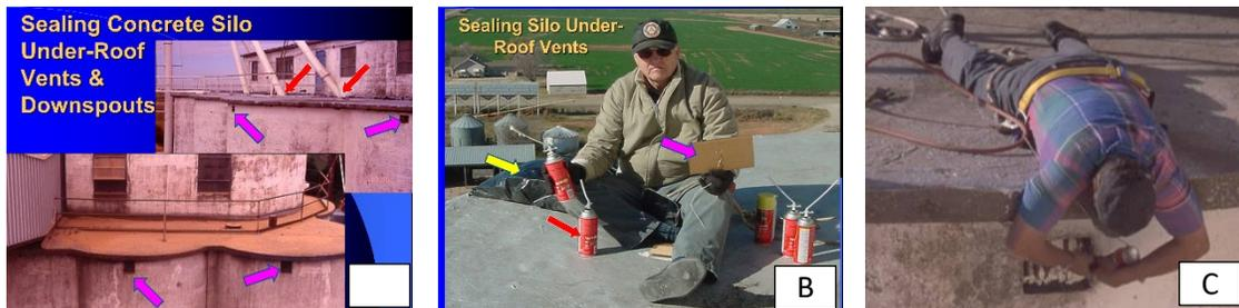
Fig. 6. Foam filling roof deck vents (A), roof vent sealing tools (B), roof vent foam sealing (C).
