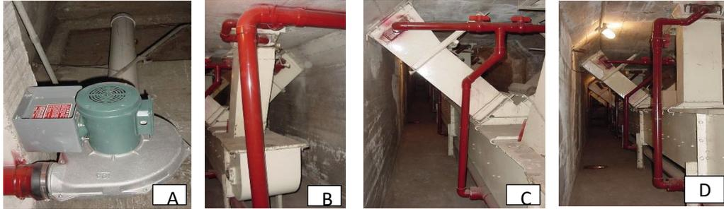
Fig. 8. CLF blower in silo annex (A), pressure manifold (B), lateral pipe to side silos (C), lateral pipe to center silos (D).
