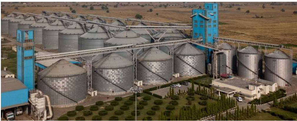
Fig. 4. Modern silo facility at Moga, Punjab.
