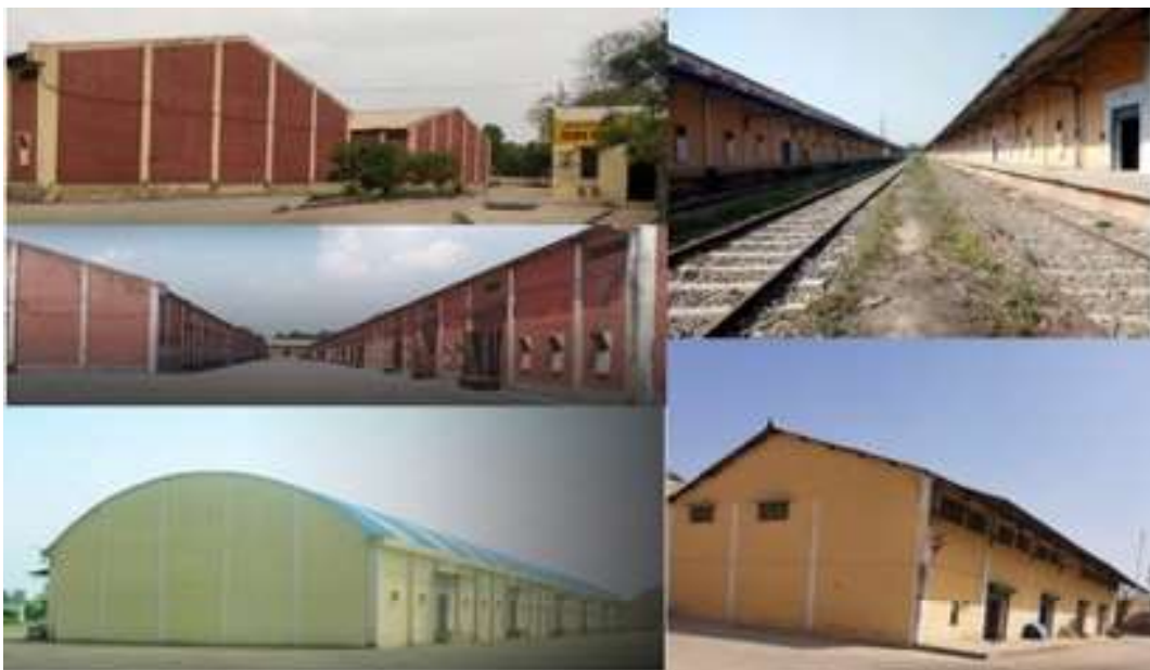
Fig. 2. Types of conventional warehouses (top and middle left); Modified single span with common road loading-unloading and with rail loading-unloading (top right); Dome shaped single span (bottom left); Gable shape single span (bottom right).
