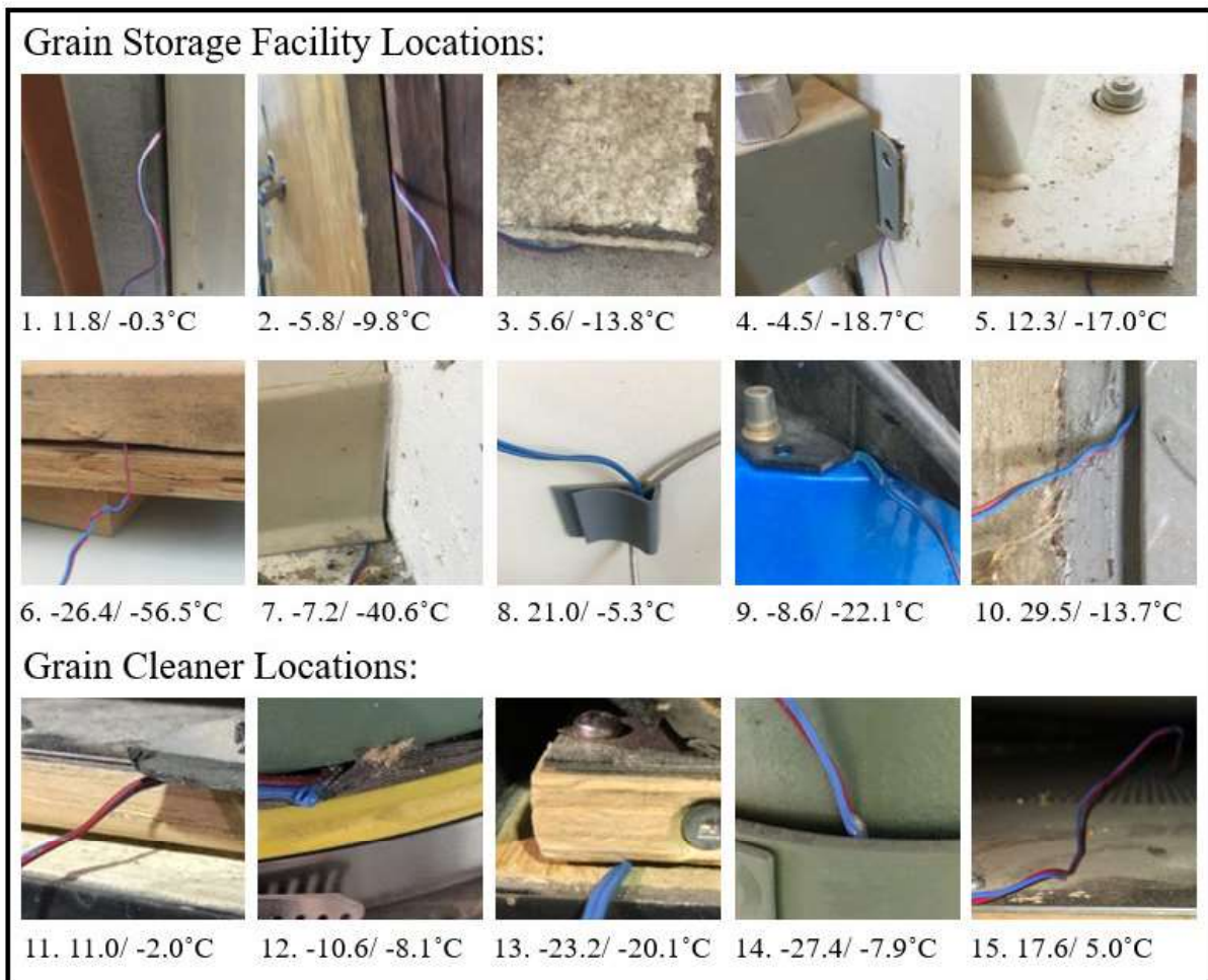
Fig. 2. Locations in Storage Facility with the minimum temperature reached on the two trials: 1. Column with two metal plates bolted together; 2. Inside of drawer on wood cart; 3. Between concrete floor and metal bin footing; 4. Between metal electrical box and drywall; 5. Between concrete floor and metal bin footing; 6. Between a piece of plywood and a wooden block; 7. Behind vinyl baseboard in corner of concrete post and drywall; 8. Inside of plastic clip used to secure small wires; 9. Corner of metal machine where 3 pieces of sheet metal are secured via bolts; and 10. Diamond plate floor access hatch. Locations in Grain Cleaner: 11. Between rubber flap and metal; 12. Between ribbed plastic and metal; 13. Between two pieces of plywood; 14. Along edge of small access hatch to metal chute; and 15. Between layers of sieves, approximately 30 cm away from spray edge.
