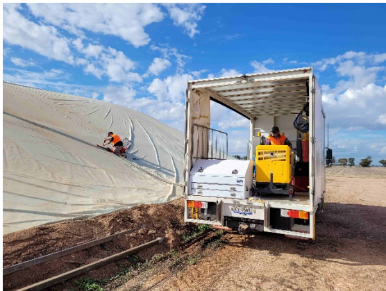
Fig. 2. Installing UltraPhos dispensing hose.
