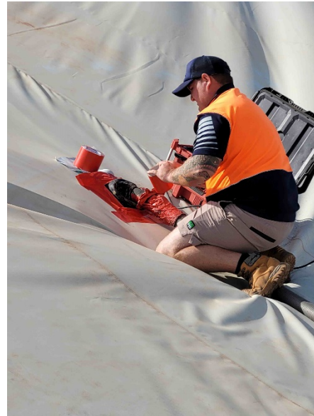
Fig. 3. Installing UltraPhos dispensing hose.
