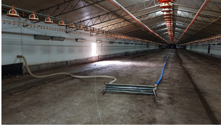
Fig. 3. Setup of the gas distribution system using a 10 cm diameter lay-flat plastic hose.
