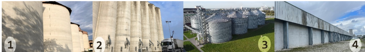
Fig. 3. Four treated storage systems located in France: 1–Baziège, concrete bins, durum wheat, no active diffusion or recirculation; 2–Roncenay, conical bottom concrete silos, peas, active gas diffusion with recirculation; 3–Pomacle, metal bins, wheat, active diffusion, no recirculation; and 4–Buchères, ground sheds, wheat, injected gas, no recirculation, and no tarping.
