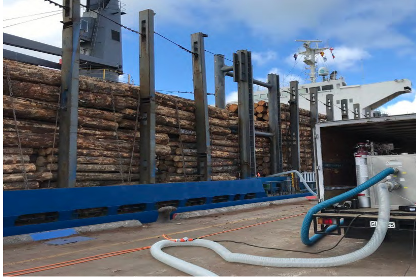
Fig. 3. Closer view of the HDS800, VAPORPH 3 OS ® , and nitrogen cylinders inside a truck.
